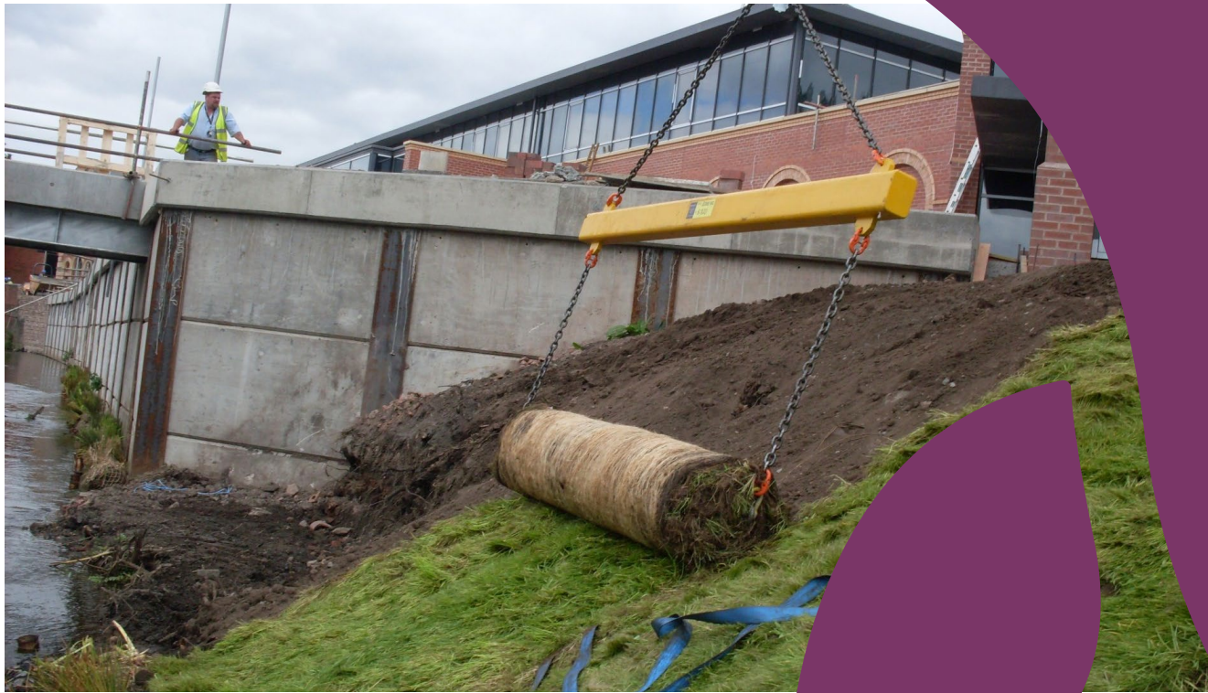
Shear Stress Turf being installed
