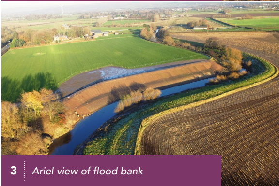
3 VMax C350 installed for flood protection
