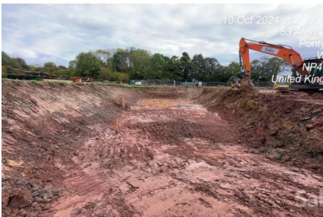
Salix was responsible for constructing the wetland cells and all associated hydraulic infrastructure, including inlets, interconnecting pipework, headwalls, outlet structures and access provisions. Earthworks were undertaken to create carefully profiled shallow basins designed to optimise retention time and hydraulic efficiency.
