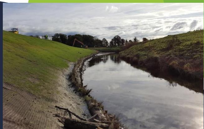
The flood bank was given the additional protection of VMax C350, this was laid over the seeded banks. This product protects the banks from shear stress, so should the area face further severe flooding the matting will ensure soils are protected and the flood bank is maintained. The VMax also benefits the banks by protecting the seeds underneath, warming up the soils and ensuring that the seeds do not get washed away in the rain or from further flooding.
