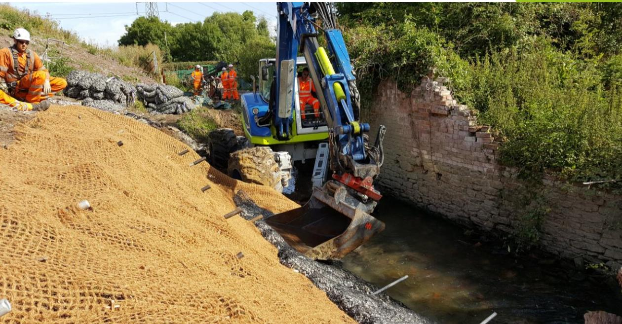
Historic undermining of the toe of the embankment on one side of the track by the river posed a particular problem.
