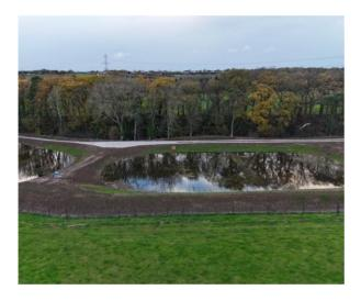
ICWs are designed to improve water quality, specifically by maximising phosphorus reduction through targeted planting. The three cells form a progressive treatment chain, with increasing depth bands and species mixes to optimise contaminant removal.
