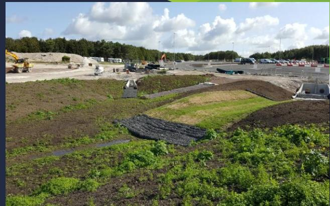
The Rock Mattresses will also prevent scour within the hydraulic jump zone of the spillway. The spillways within the detention basin are covered with Shear Stress Turf (SST) that protects the engineered soil and clay lining beneath. Shear Stress Turf is a unique pre-vegetated scour solution typically used in areas where forces exerted by water exceed the shear limits of other Turf Reinforced Mats from day one of installation.
