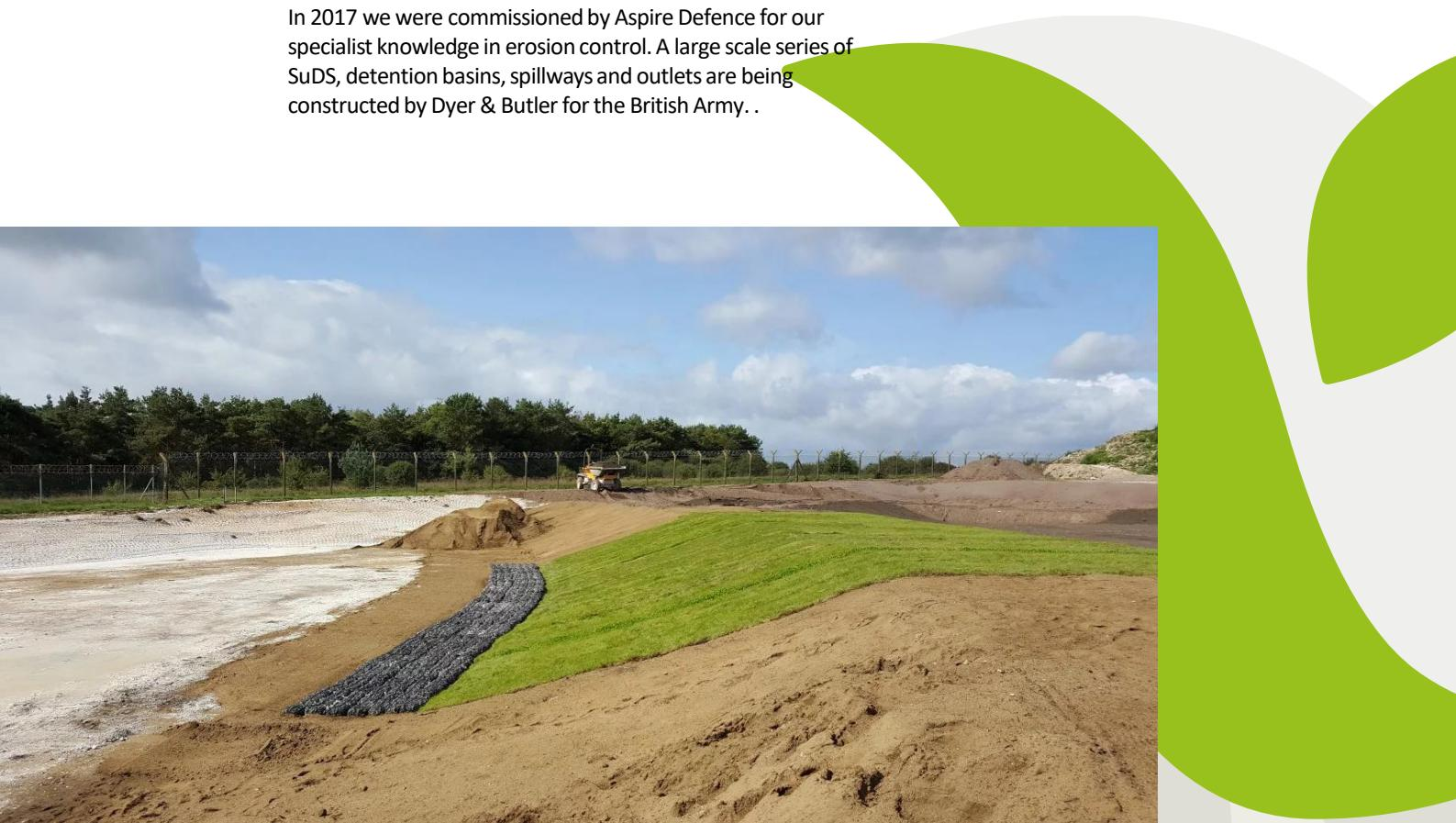
Aspire Defence, the design engineers, made particular use of three of our erosion control products, including Rock Rolls, Rock Mattresses and our Shear Stress Turf.
