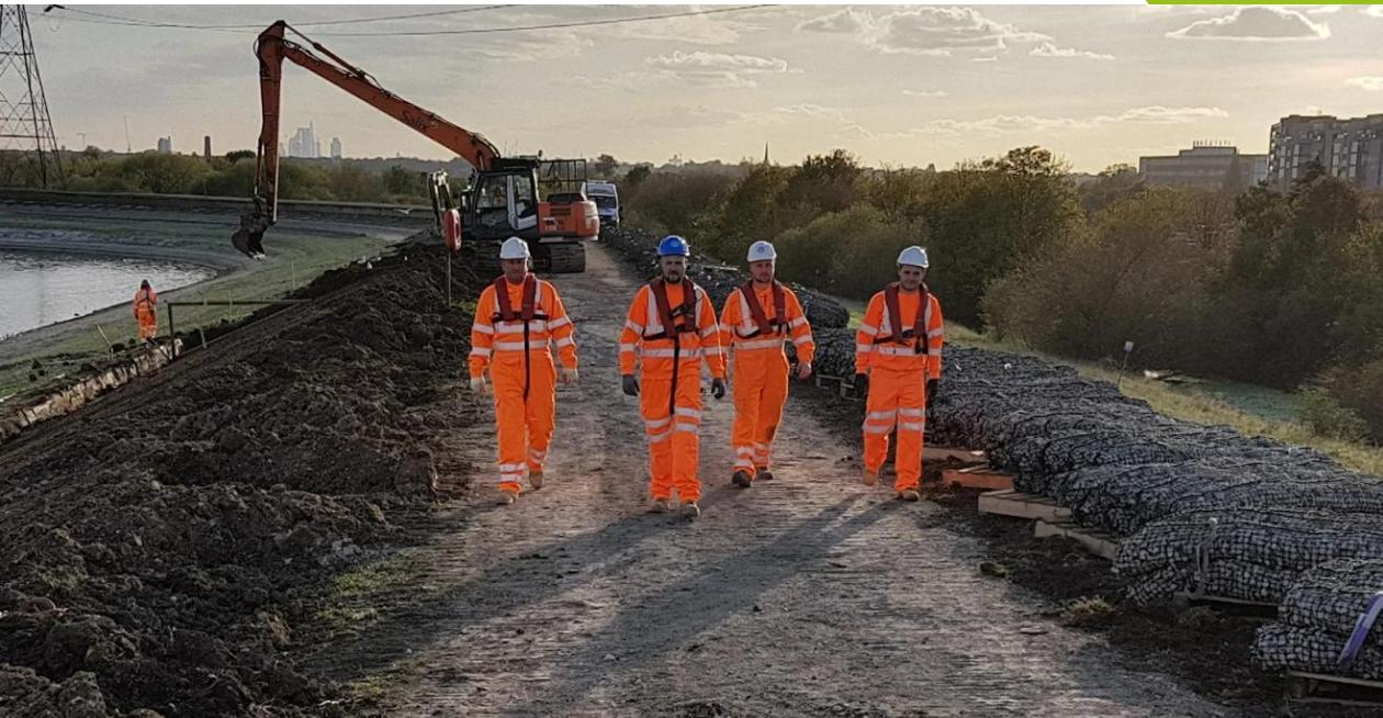
Salix have completed a project on a reservoir in North London to provide a sensitive solution to erosion issues along a stretch of the shoreline. The reservoir, which has a crest length of around 2,670 m is impounded behind an earth fill embankment dam which has a puddle clay core at its centre.
