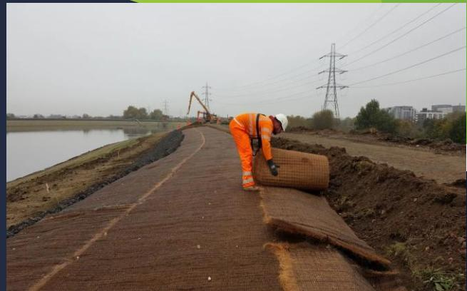
The prefilled rock mattresses offer a robust engineering solution to the erosion problems but also provide an environmentally beneficial outcome by using small stones that accrete sediment, encourage vegetation to establish and provide invertebrate habitat within the stone.
