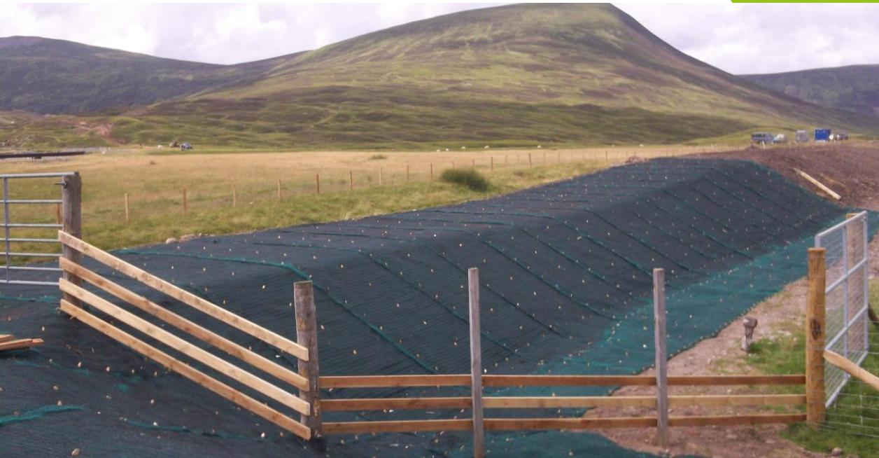
VMax<sup>3</sup> P550 is composed of a permanent, ultra-high-strength, three-dimensional matting structure incorporated with a permanent 100% polypropylene fibre matrix. This is the highest performing TRM (Turf Reinforcement Mat) in the world, providing long term erosion protection and vegetation establishment assistance while permanently reinforcing vegetation. P550 is designed for use on steep slopes, high-flow channels, spillways, and shorelines.
