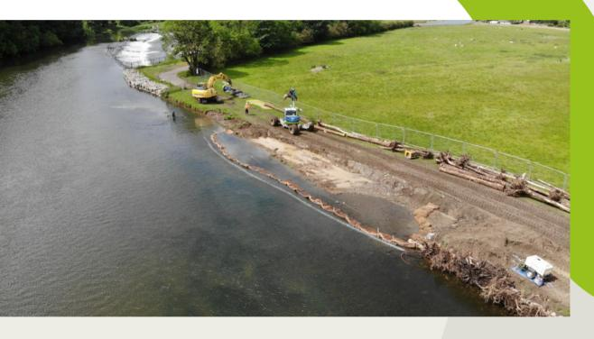
Erosion processes during flood events were twofold, firstly severe bank erosion caused by toe scour, bank failures and associated bank retreat and secondly the stripping back of the turf layer on the flood plain, exposing further floodplain soils to erosion. The river also began to cut a new channel on a shorter course across the floodplain, bypassing a large weir structure, a process known as avulsion.
