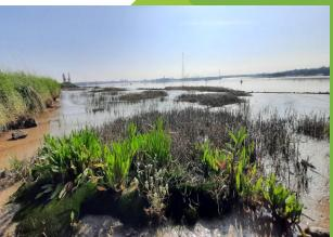
The project encompassed 600m of eroding saltmarsh and the design made use of brushwood fascines as a biodegradable method to retain sediment, whilst allowing water levels to rise and recede unimpeded.
