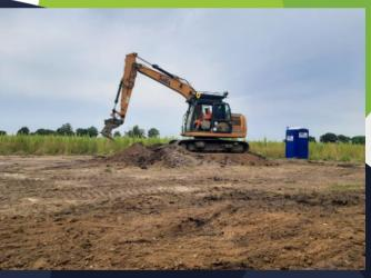
Sedi-Mats and silt wattles were used to reduce the impact of sediment migration and preserve water quality during the works. Track matting was laid to ensure safe access for heavy machinery without causing soil compaction or erosion.
