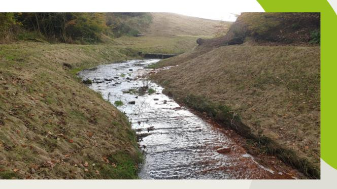
The Environment Agency have decommissioned two reservoir dams at Jack's Key and created an engineered channel between them that feeds into the River Darwen.
