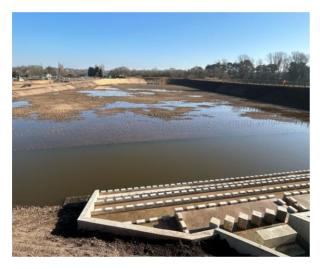
In addition to the pre-cast structures there are cast-in-situ cascade steps, gabion baskets and rip rap to install at each of the inlet / outlet structures.
