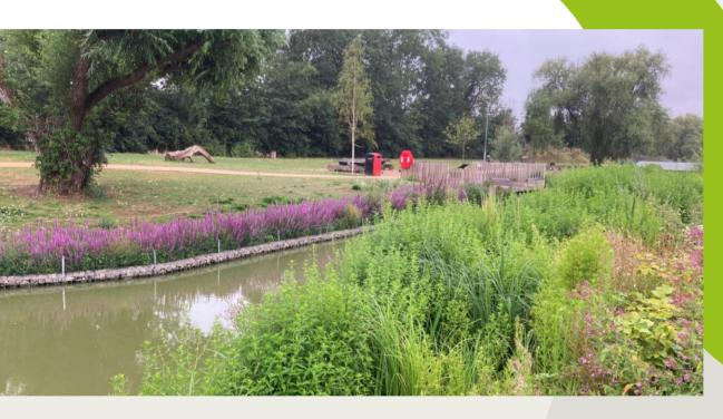
Salix worked with the designers, HTA, to provide a solution, which consisted of creating marginal habitat shelves. New banks were formed within the pond using a retaining feature, with a finish level very close to the water level. Pre-established coir pallets were installed on the new shelves, which provide mature vegetation to rapidly speed up the establishment and increase habitat.
