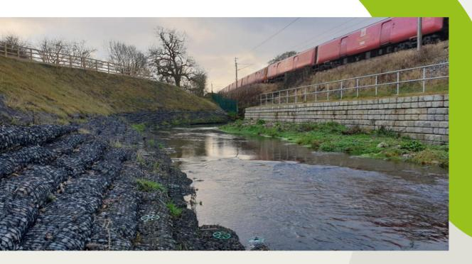
The solution consisted of using Salix's RockLockTM – a combination of Rock Rolls and ground anchors to provide an ultimate fixing solution in high-energy environments. Given the flow velocities, ground anchors help to prevent the movement of the Rock Rolls.
