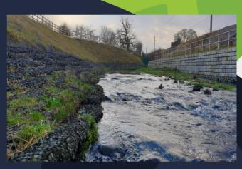
Rock Rolls and Mattresses utilise a UV-stabilised virgin HDPE net containing a 40-80mm stone. Virgin HDPE has an estimated design life of up to 100 years.
