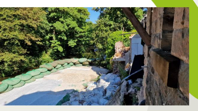
Jackson Civil Engineering approached Salix to supply over 500 pre-filled two-tonne AquaRockBags to use as immediate flood protection, and the bags were reused later as part of a temporary work piling platform.
