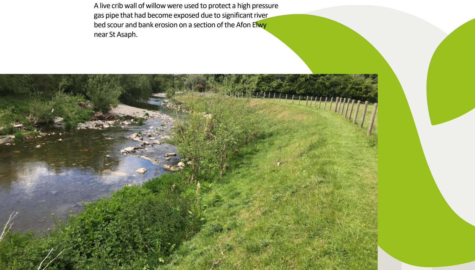
Attempts had been made previously to protect the pipeline with a large gabion structure, but this had actually accelerated the erosion problems directly over the pipe.
