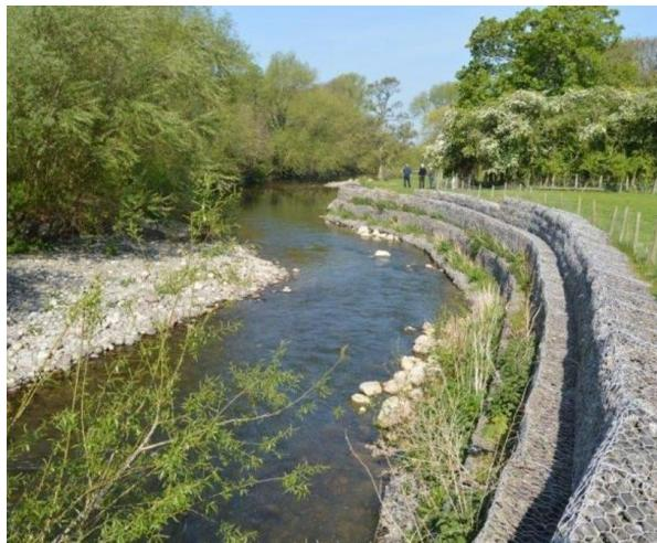
The gabions jut out into the flow and enforce a left turn, and as the gabions end, the flow separates with a shear layer, expands considerably, and causes the recirculation. The proposed design was to remove the gabion structure and re-grade the right bank.
