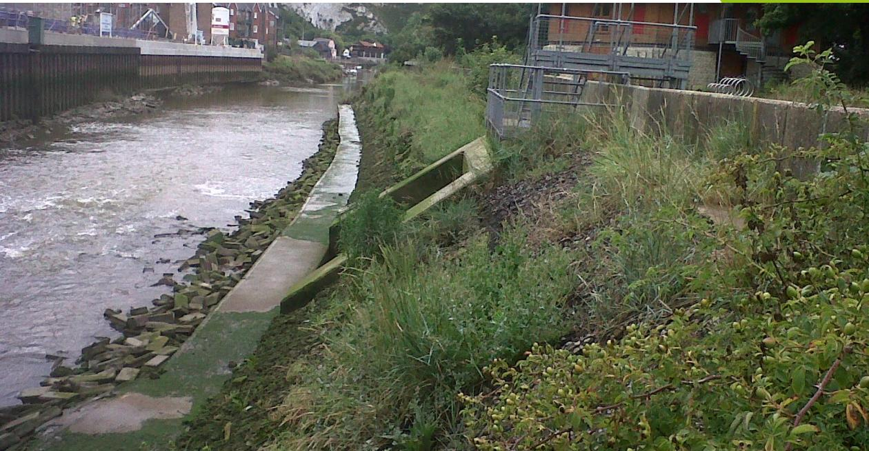
The integrity of the existing blockwork facing was deteriorating as a result of the tidal inundation and draw-down cycles together with areas of groundwater seepages emanating from the slope profile.
