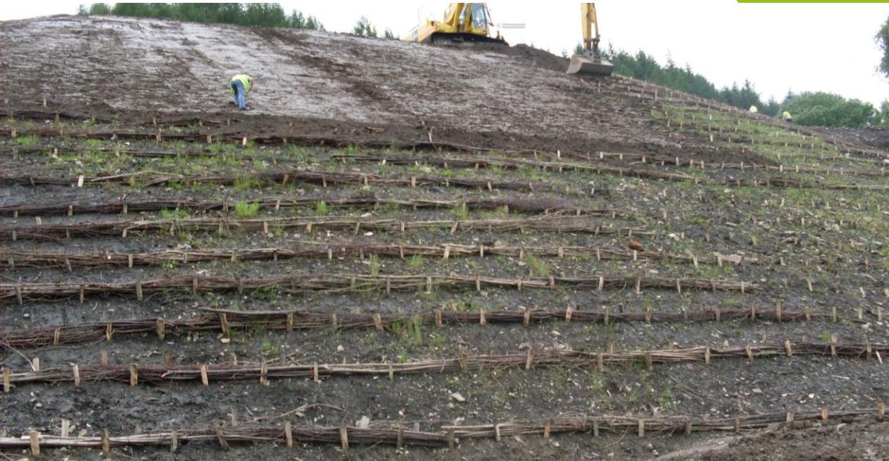
The geotechnical issues were solved using our grids. For the surface treatment, Salix installed a series of dead willow fascines at 1.5m spacing down the slope in order to physically retain the 250mm of soil cover. Willow fascines are a more environmentally sustainable alternative to cellular confinement systems and are easier to fill.
