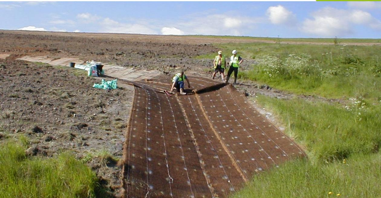
Analysis of the channels revealed that even if vegetation could be established the uncohesive sandy soils would not remain stable as the predicted flow velocities would be too extreme for a grass cover alone to withstand.
