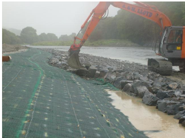
Blockstone toe with NAG above replacing blockstone
