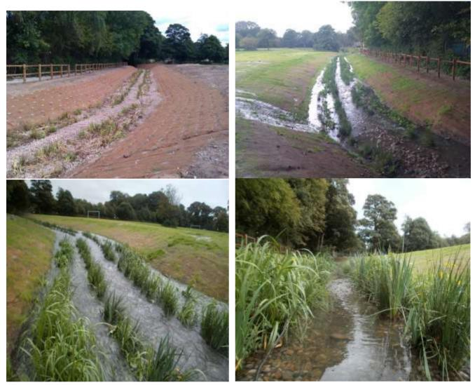
The above images illustrate the early stages of our work on site through to how the finished scheme appears today-the pre-established coir rolls are now mature.
