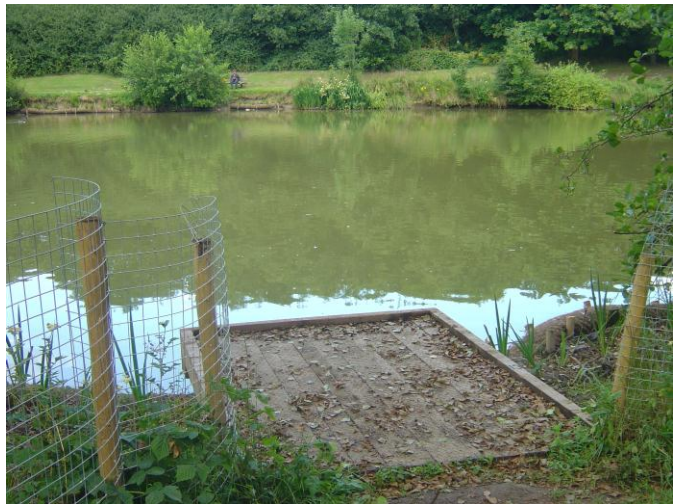
Fencing protects planting between fishing platforms
