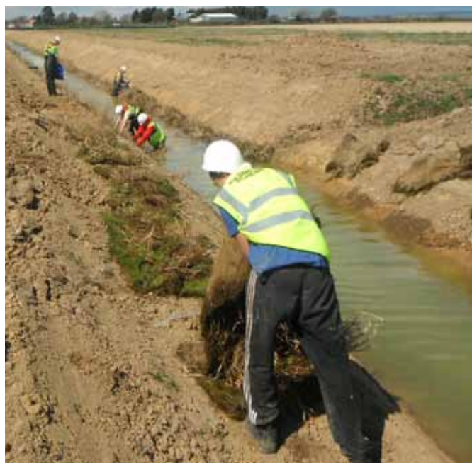
Coir Pallets installed April 2012
