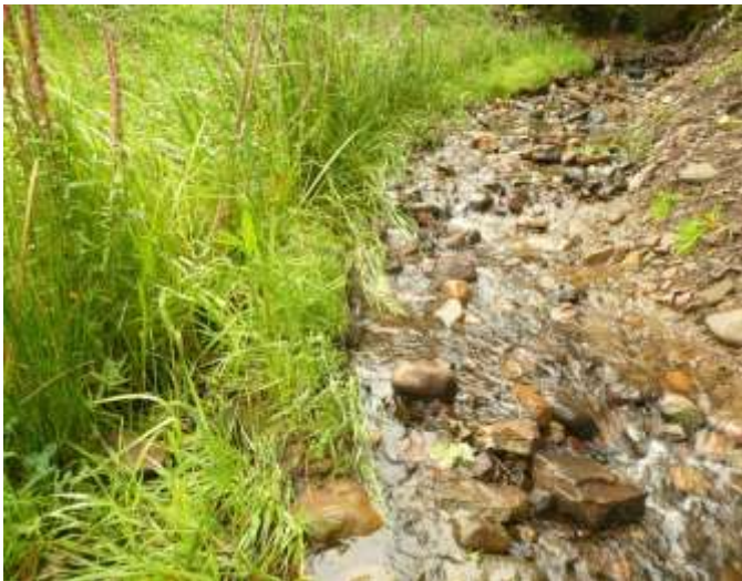
Two months after completion of works.
