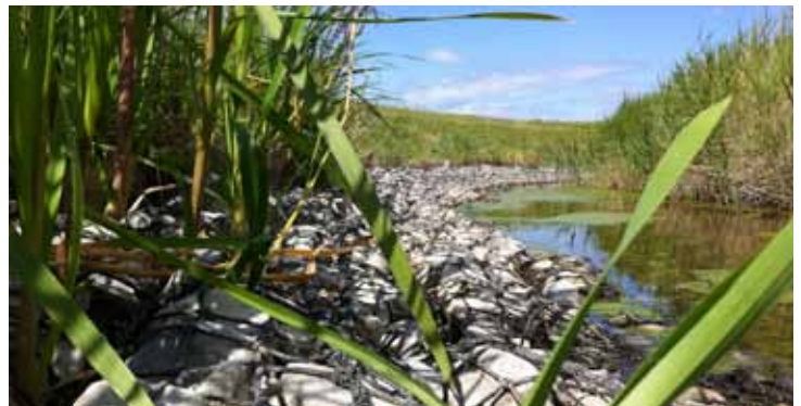
Rock Mattresses tie in detail at hydraulic jump zone with Vmax C350
