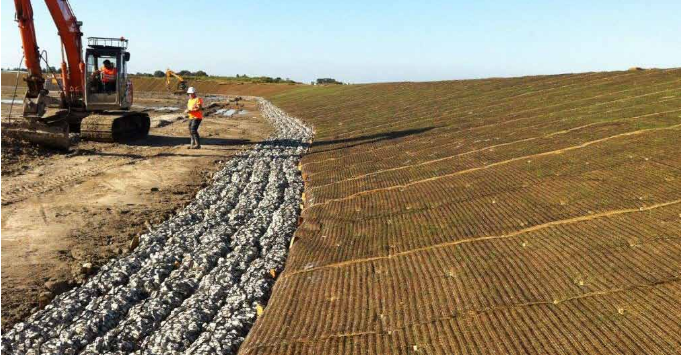
Rock Mattresses tie in detail at hydraulic jump zone with Vmax C350
