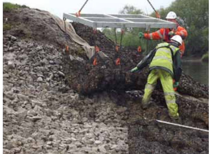
Rock Mattresses being installed
