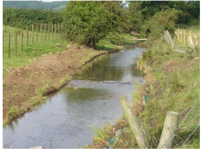
Pre-established coir rolls set into channel
