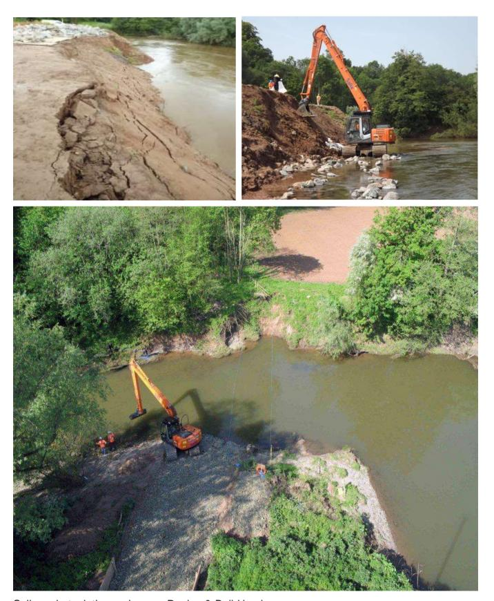
Salix undertook the works on a Design & Build basis. Innovative working methods included a submerged blockstone causeway that permitted fish movement and allowed access to the opposite bank to work.
