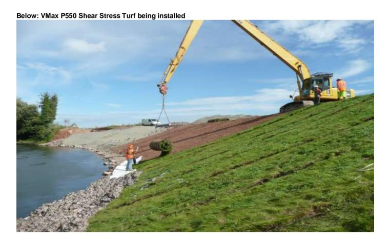
Trees limbs removed for access were reused as part of the soft engineering revetment. Salix grew in-house over 2000m2 of reinforced grass/wildflower turf on 40m2 large rolls to provide soft engineering protection above average low water level. The high erosion control performance of this turf meant that a soft solution could be used as a direct alternative to rock rip rap, saving over 1000 tonnes of imported material whilst creating a more sustainable and ecologically valuable solution.
