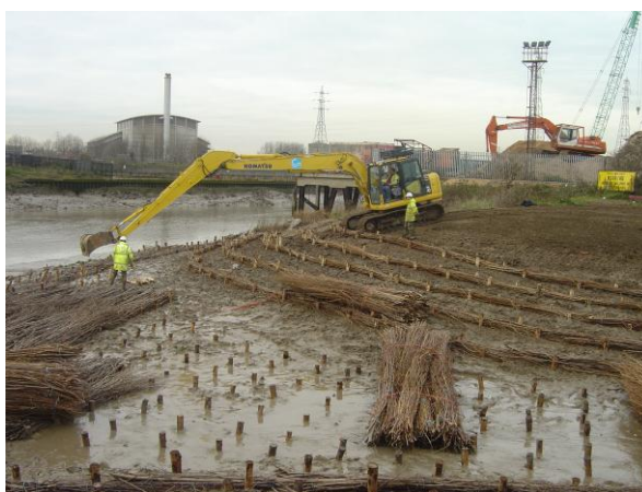
Installation of brushwood faggots
