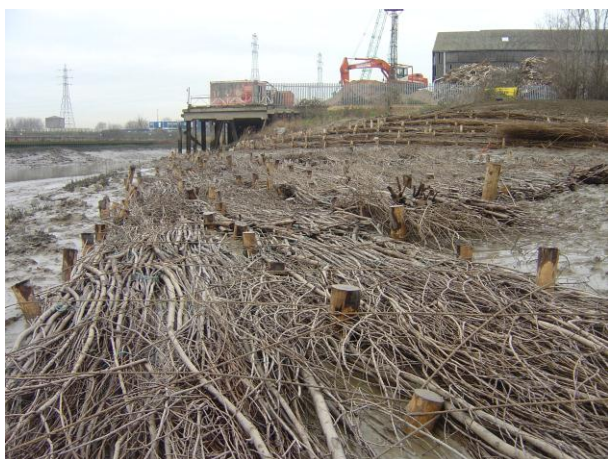
Brushwood tied down to accrete
