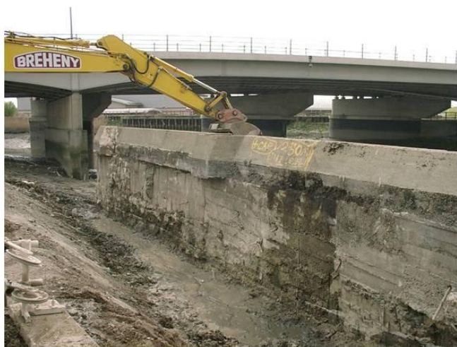
Vertical river wall removed to create natural sloping bank
