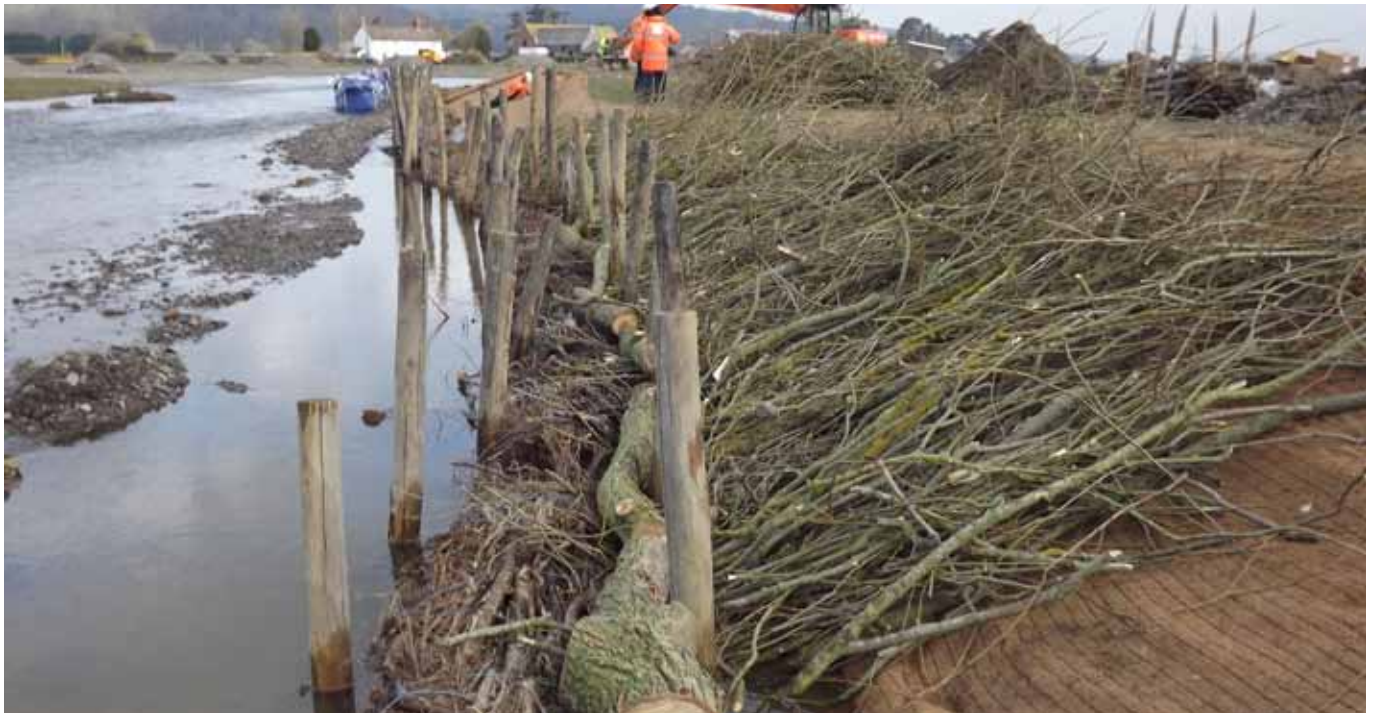
Installing a live brush mattress revetment with whole tree toe
