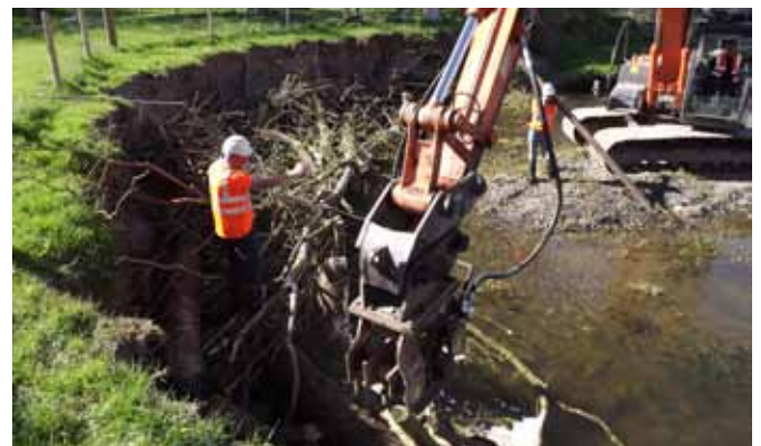
Staking branches and brush into place
