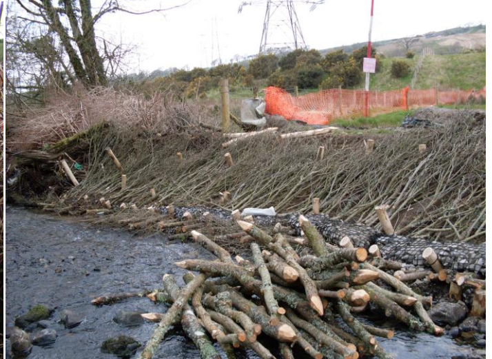
Bioengineering works during construction
