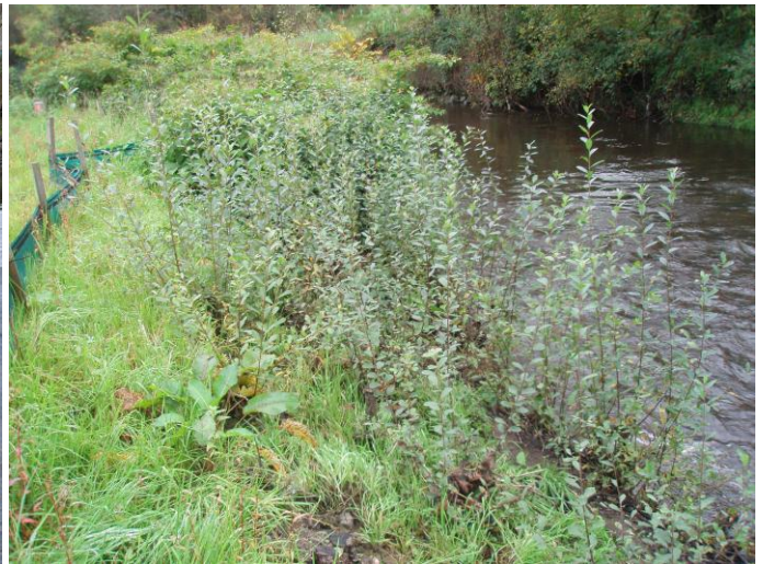
Growth of bioengineering revetment after 1 year
