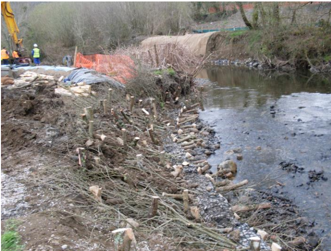
Completed bioengineering revetment
