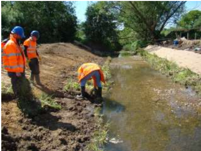
Installing pre-established coir pallets
