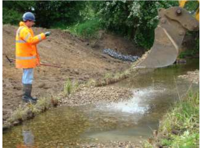
Banks graded and gravel introduced
