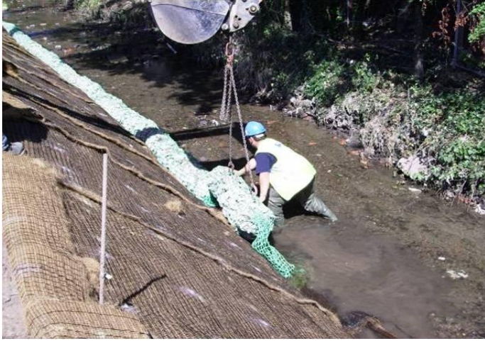
Installing rock roll toe
