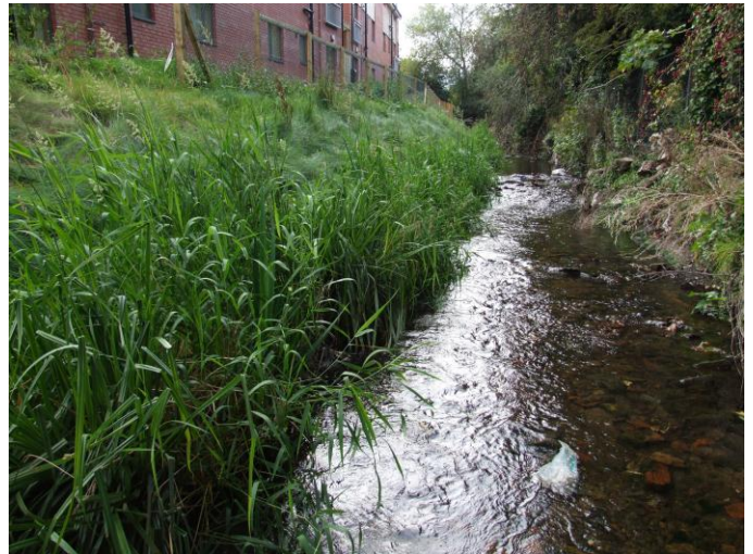
Fully established bioengineering solution
