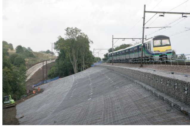
Vmax C350 under rock netting
