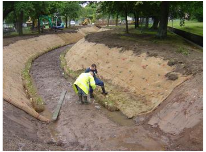
Installation of coir rolls and NAG C125BN
