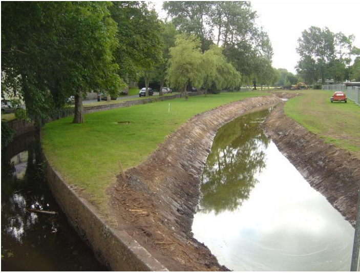
Old concrete channel next to new channel
