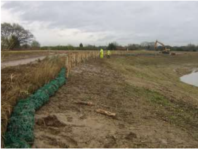
Rock Roll and Coir Roll Revetment Installation.
