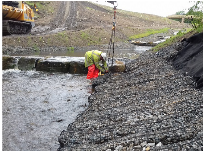
Rock Mattresses being installed
