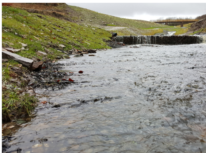
Rock Mattresses through bed of channel and along the sides blending in well shortly after installation
