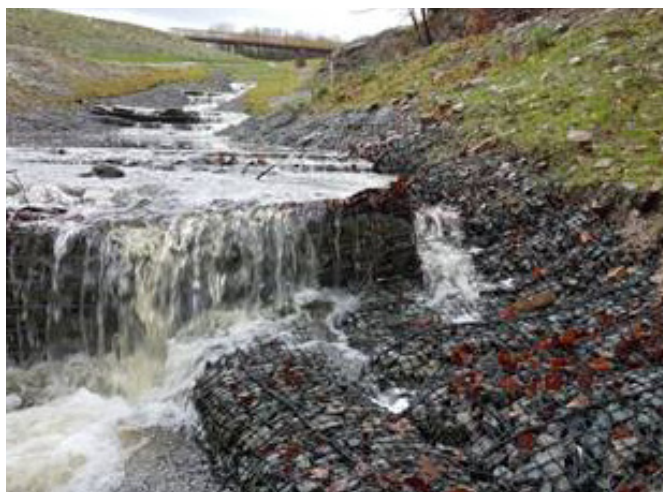
Looking upstream. Salix pre-filled Rock Mattress shaped and placed around the failing gabion mattresses. The flow now stays within the channel and on top of the Rock Mattress with its tighter stone fill.
