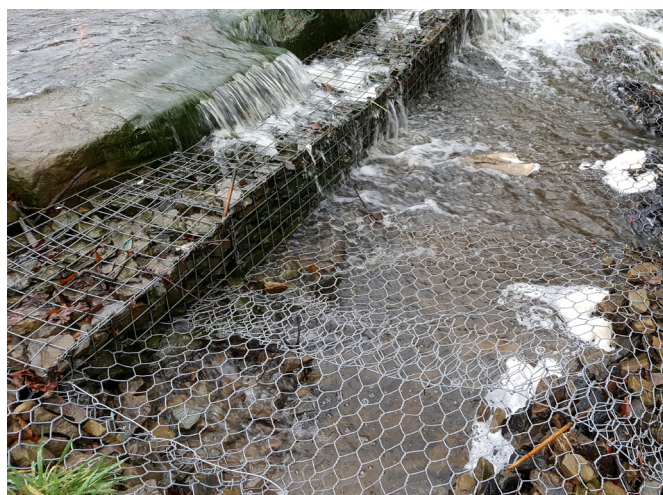
Due to high energy water flows the stones within the gabions have moved leaving large voids
