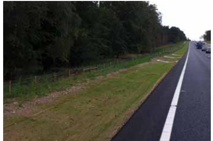
Rapid establishment of grasses shortly after installation
