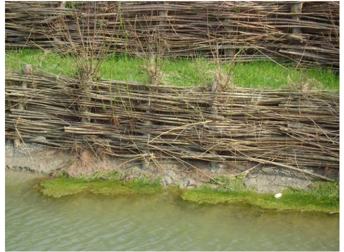
Close up of spiling
