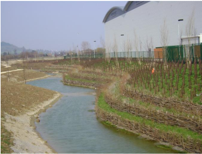
Newly installed Willow spiling
