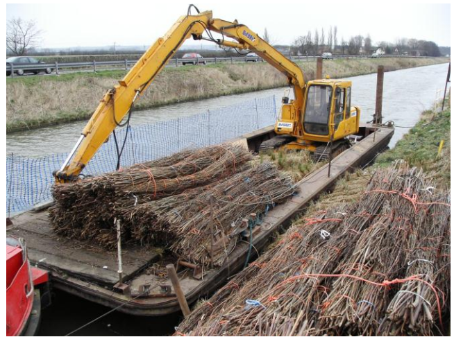
Brushwood faggots delivered by barge
