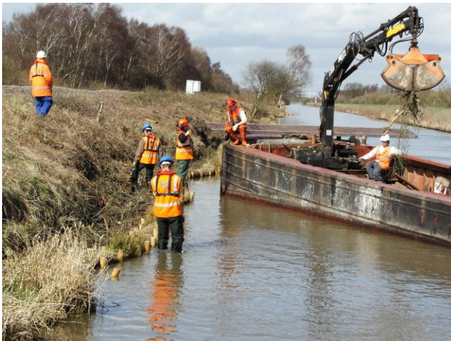
All works from barge access
