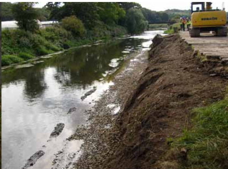
Stone is used as backfill up to average summer water level. Locally won soil is used above this level
