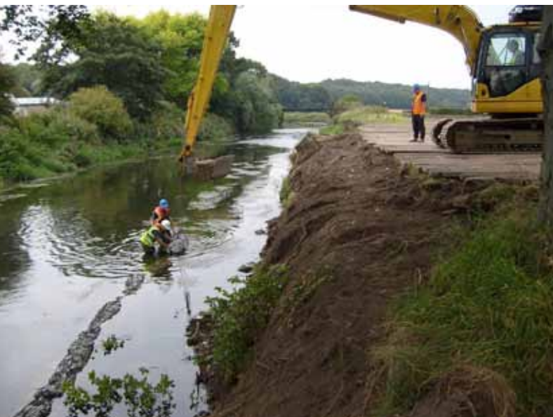
Rock Rolls are installed to create a toe revetment and also to act as a coffer dam to prevent sediment release from the bank works.
