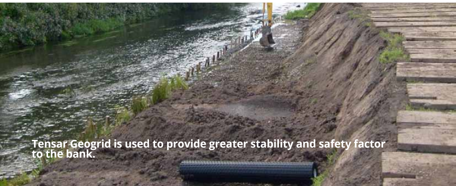
Rock Rolls are installed to create a toe revetment and also to act as a coffer dam to prevent sediment release from the bank works.
