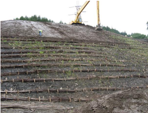
Installation of willow faggots
