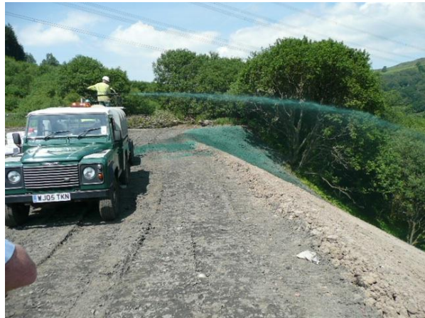
HydraCX applied over finished surface
