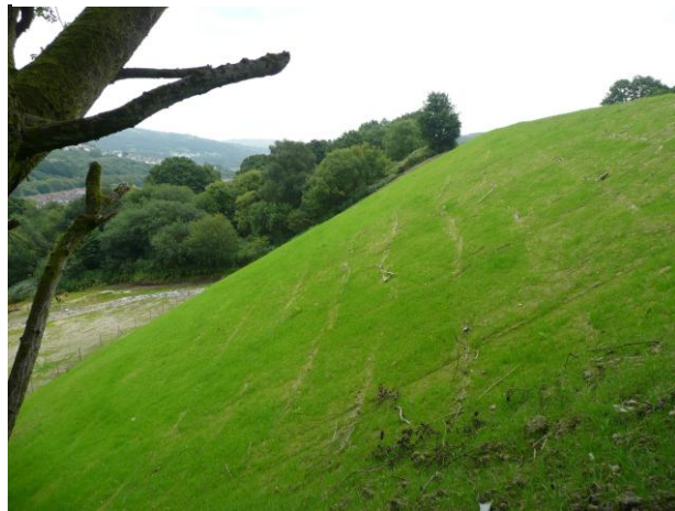
24 days later after severe rain events
