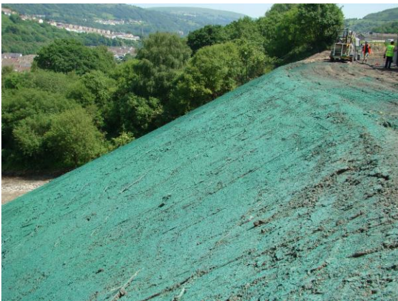
Day after installation of HydraCX
