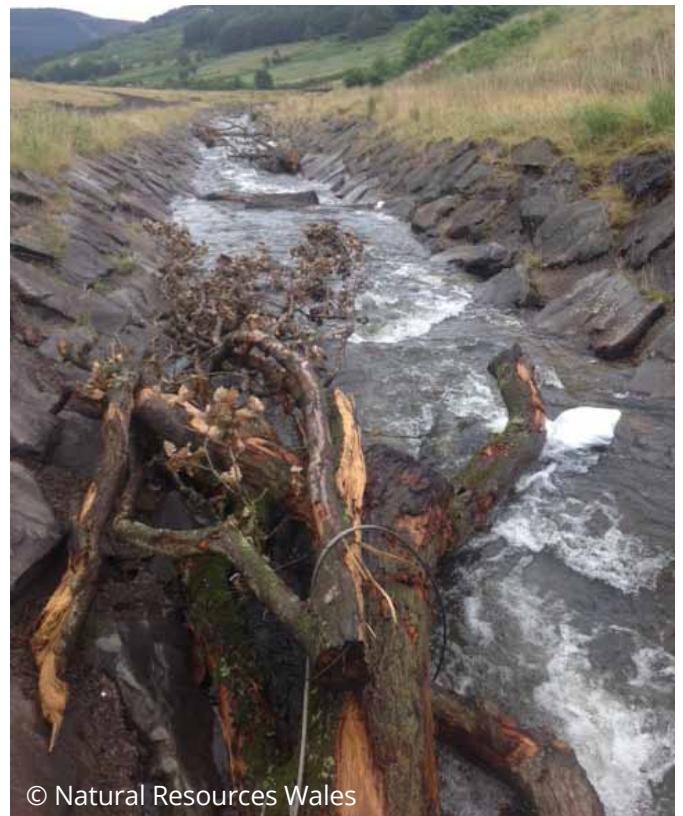
Large woody debris tied onto the stream bank
