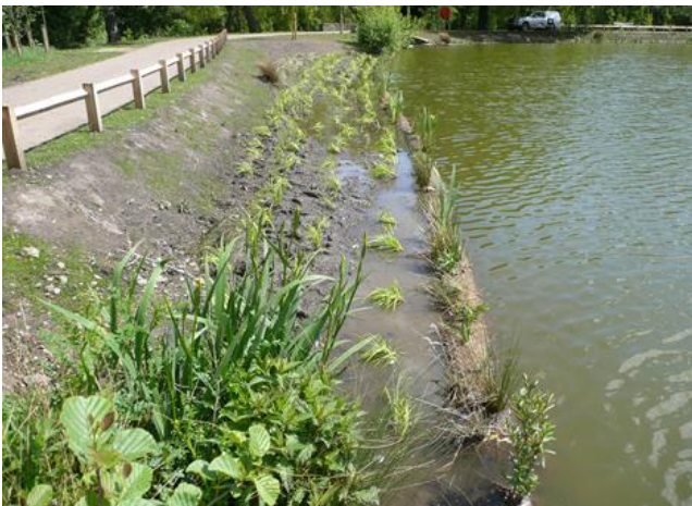
Newly installed Coir rolls and wetland planting
