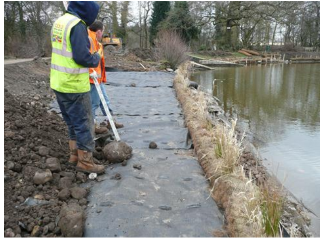
Coir rolls placed onto woven geotextile and backfilled
