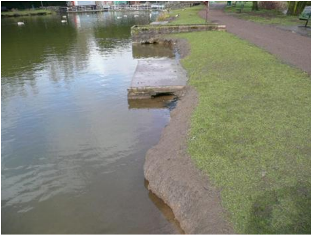
Typical state of lake edge prior to works
