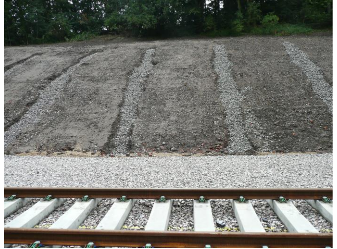
Final profile with drainage
