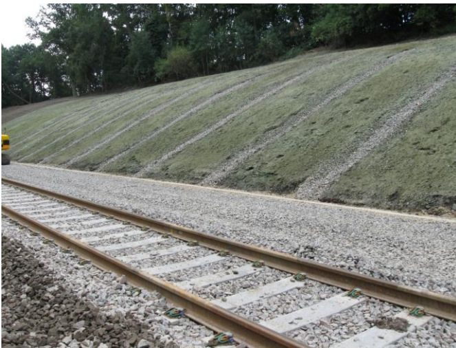
Immediately after applying HydraCX
