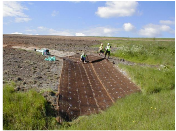
Vmax C350 manually installed
