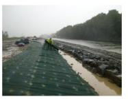
Unprotected seed and soil are highly susceptible to erosion. Upon installation, the P550's polypropylene fiber matrix and corrugated matting structure provide a uniform mulch layer and effective erosion protection for seed and soil under flow-induced shear stresses up to 191 Pascal or up to 3.8 m/s flow velocity.
